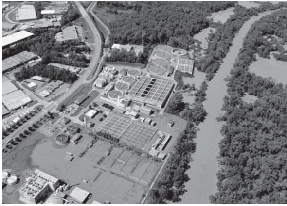
Atlanta's R.M. Clayton Plant flooded during September storm.
